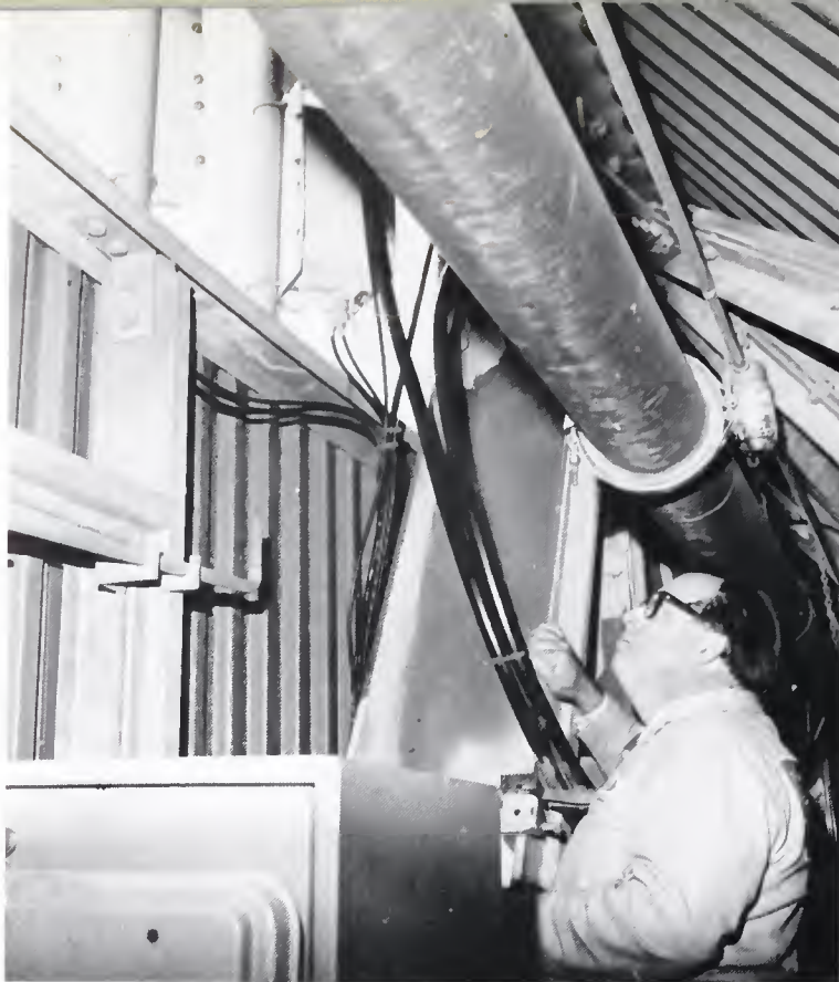
Figure 3. Nurad ENG pickup horns are mounted on the 4th level. Catwalks are sheltered up through the 4th level to protect equipment and permit all-weather access. Specific antennas are selected by remote control from the downtown ENG control point. Signal is down-converted to 70 MHz IF and piped down to equipment room over coaxial cable, as with point-to-point links.
