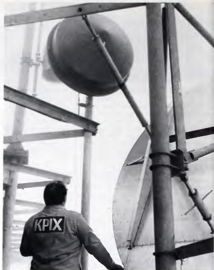
Figure 5. Protected dish on the 2nd level, some 1020 feet above sea level, receives 13-GHz signals from Mt. San Bruno. Passive reflector on right is from some other service.
