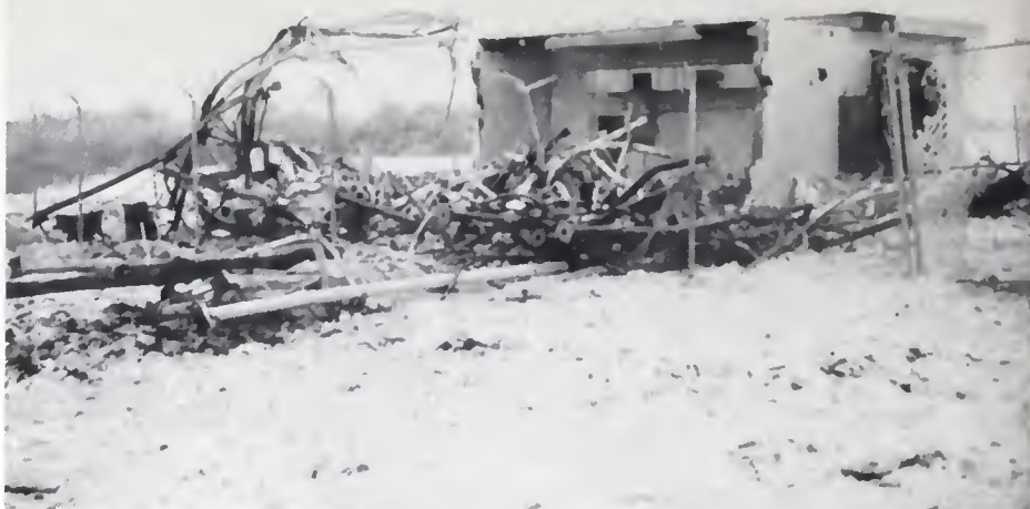
Two-thirds of the Channel 14 transmitter building was completely pulverized by one or more tower sections having fallen on it.
